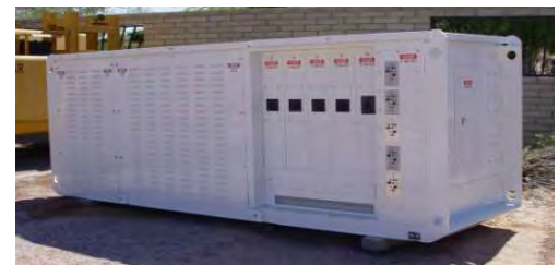
15kV Transformer
