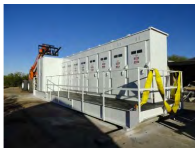
Skid-Mounted Switchgear
