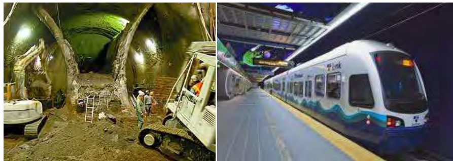
Beacon Hill Tunnel and Stations
