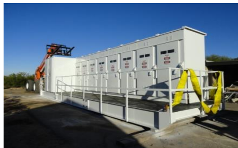
Skid-Mounted Switchgear
